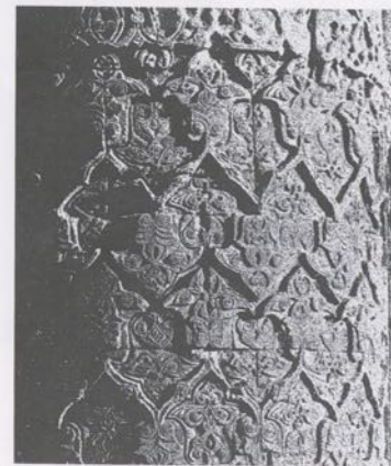
Sivas, Gok Medreseh, southwest corner of Blind Tower
